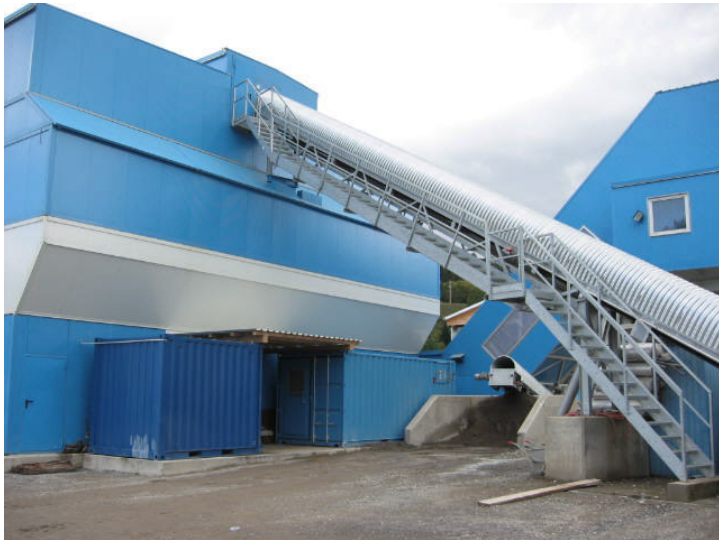
The aggregate silo with the Turbomatic thermal energy unit
